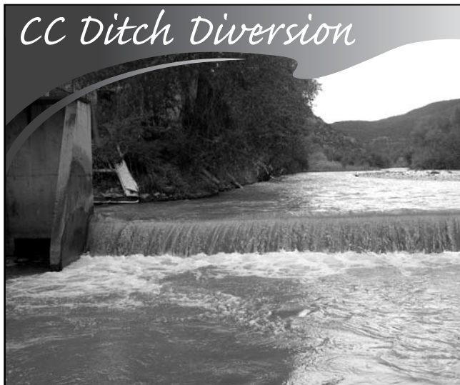
Fish ladder construction scheduled for 2011.
