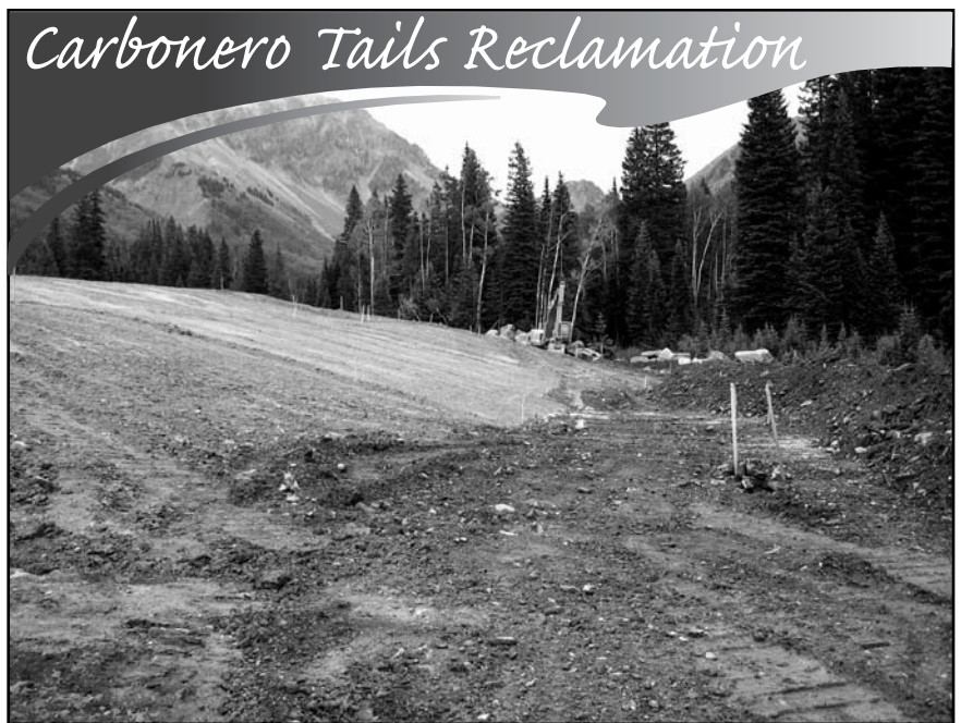
Tailings were moved away from Howard Fork floodplain, graded and capped.
