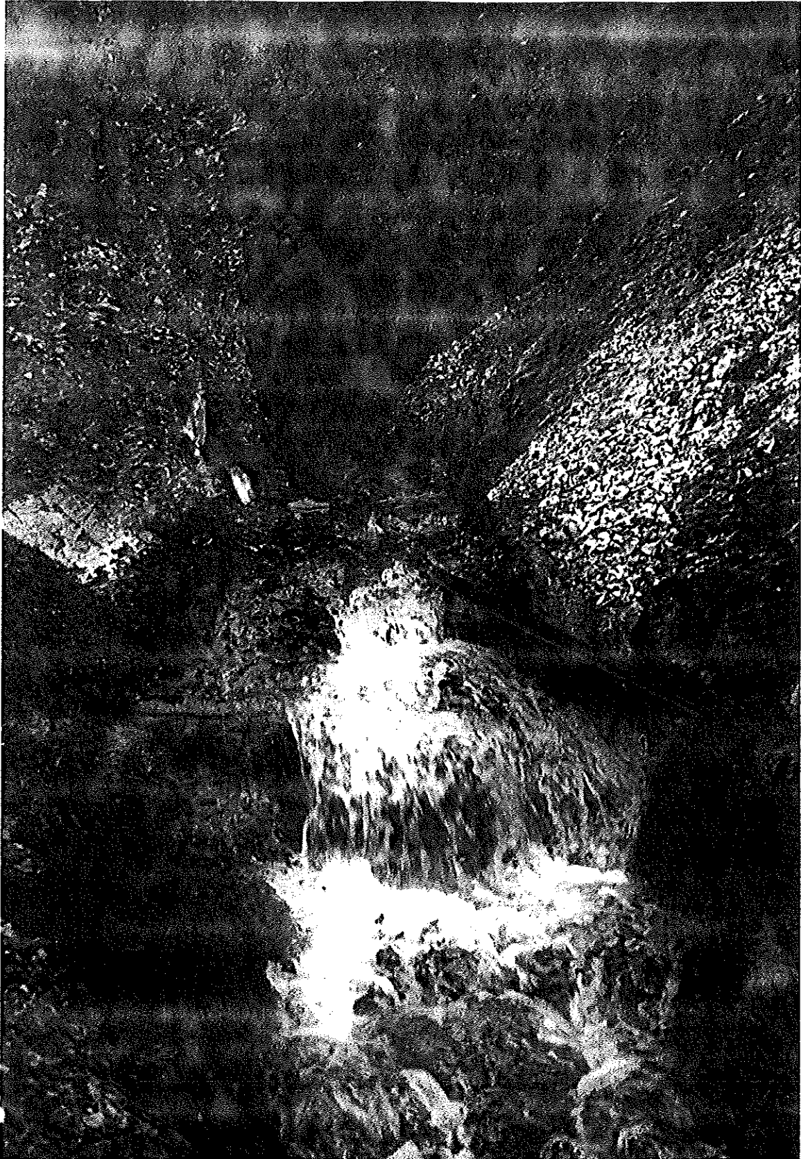
Figure 9. Portal, effluent, and terracettes of precipitate at adit #101.
