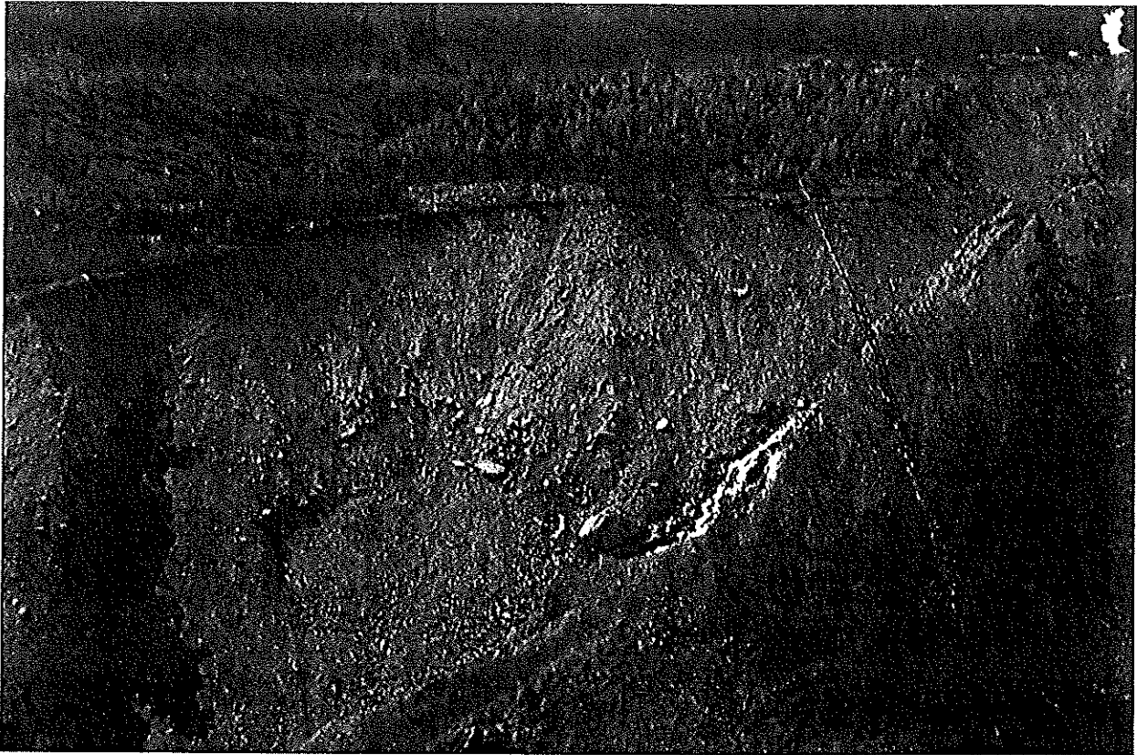
Figure 23. Severely eroded gulch below the Carbonero Mine (inventory feature #104).
