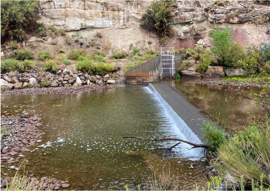
Figure 10. Reed-Chatfield diversion dam.
